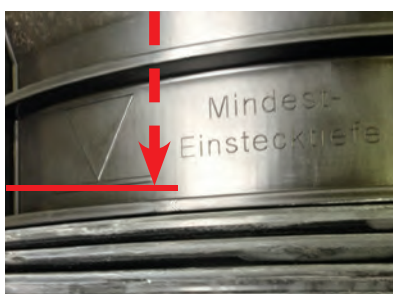
Insert to at least the minimum depth!
