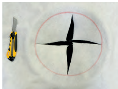
Cutting a cross within the marked circle
