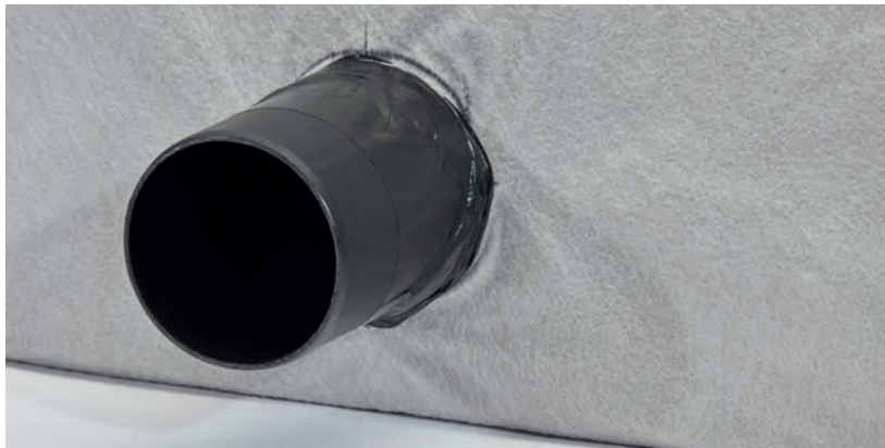
The geotextile is cut in and is pushed over the pipe adapter
