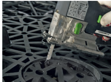
A keyhole saw with extra-long saw blade is required to cut out the pipe connection opening in the side panel
