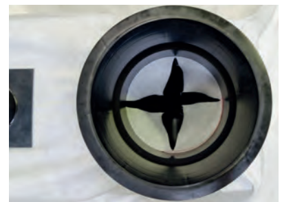
Installing the intermediate section (= sand tight)
