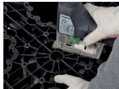
A keyhole saw with extra-long saw blade is required to cut out the openings for the pipe penetrations in the side panels and at the top of the basic elements
